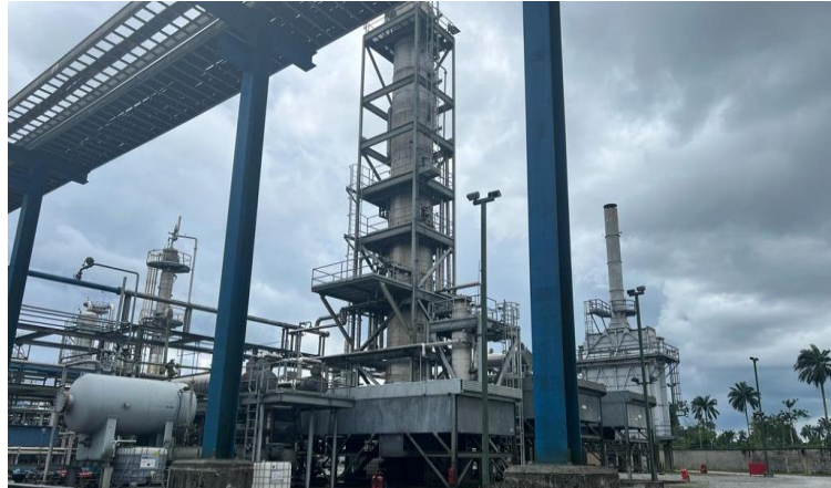
Modular Refinery Train 2 at 5000 bbls/d capacity
